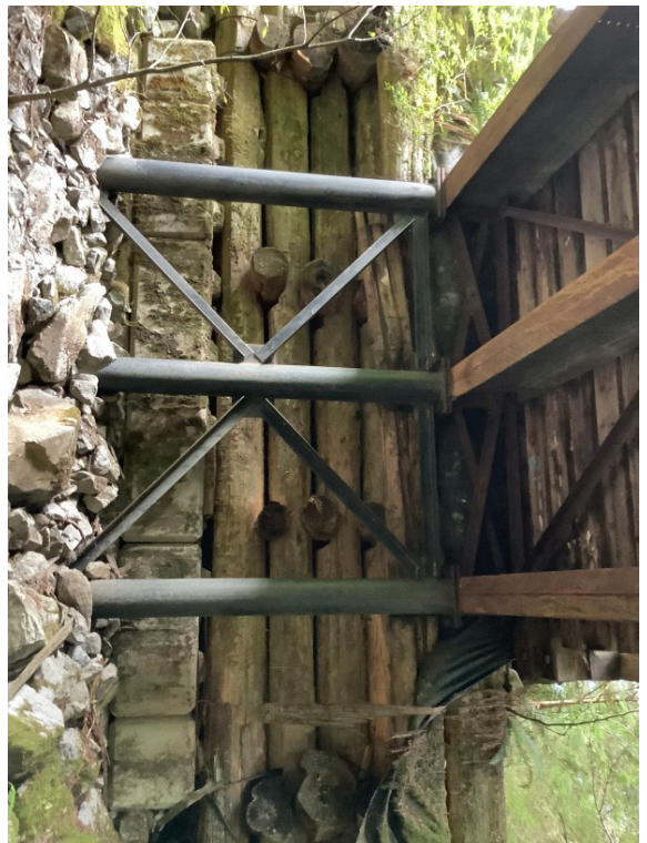
Right Bank Abutment when facing downstream
