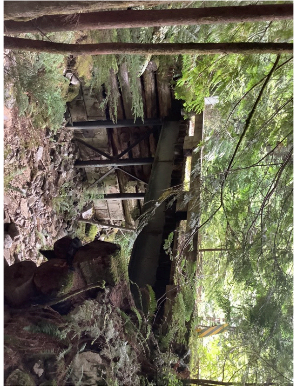
Left Bank Abutment when facing downstream
